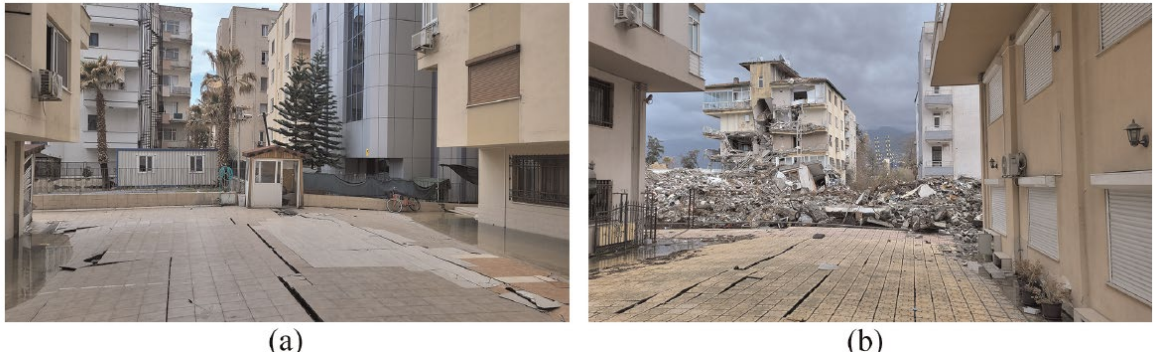
Figure 2-20 Hogging in the courtyard of four buildings in Area 1: (a) facing west with Building G on the left and Building J on the right; (b) facing east with Building I on the left and Building H on the right (from Moug et al., 2024).
