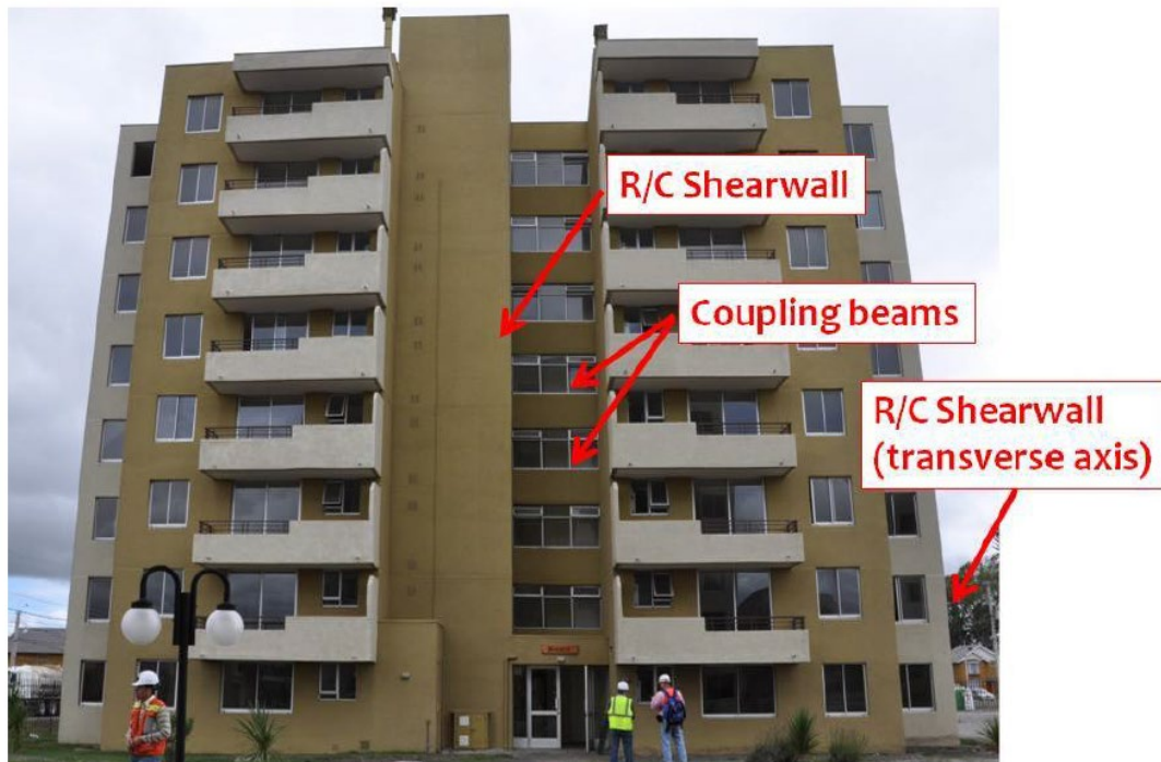
Figure 2-12 General components of the structural system in Riesco Building (from Bray and Frost, 2010).
