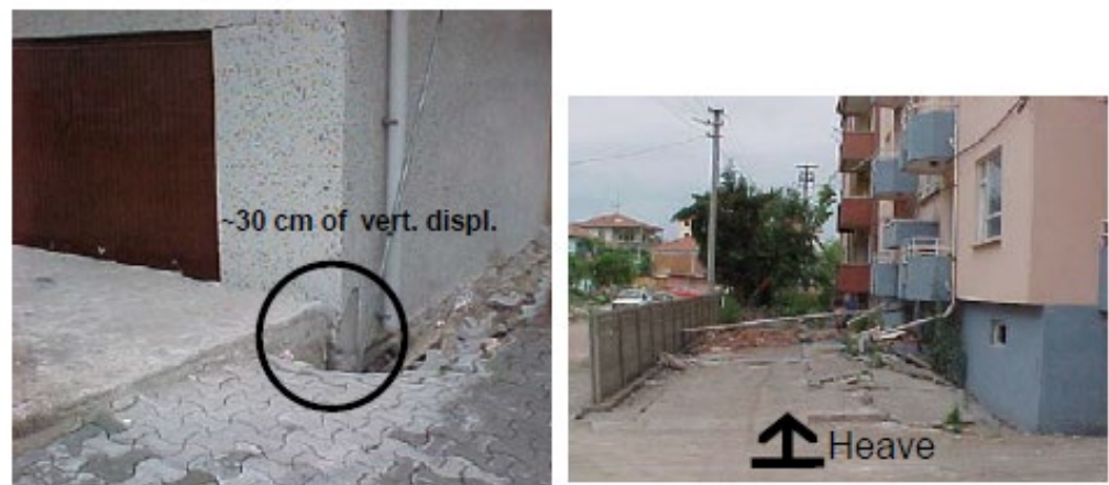
Figure 2-6 Examples of vertical displacement and heave observed in Adapazari after the 1999 Kocaeli earthquake (from Bray and Sancio, 2009).
