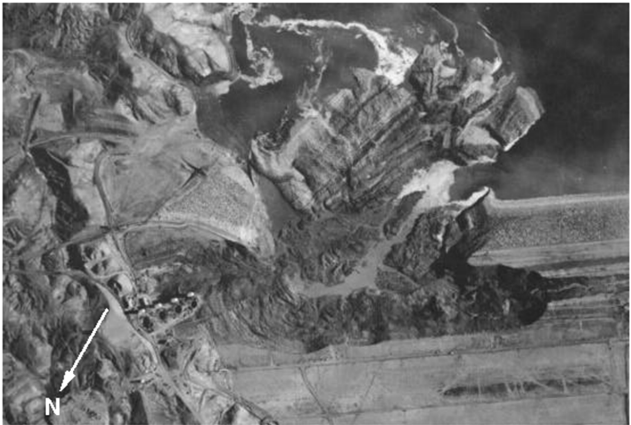
Figure A.2.2: Enlarged aerial photo from Figure A.2.1 showing failure at the east end of the dam. (from http://www.midrivers.com/~rafter/lake/ )
