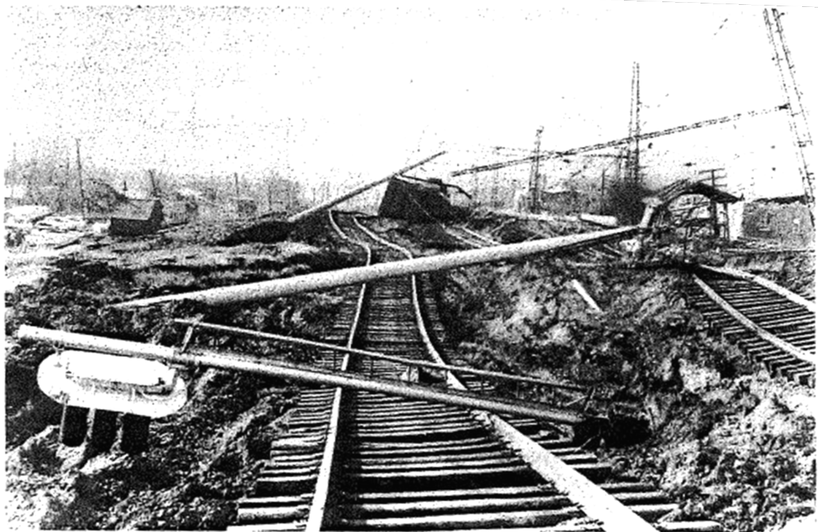
FIG. 13. Photograph of Failed Embankment at Railway Station in Nalband (Site 3) (Photo Courtesy of A. Karakhanian, 1989)
